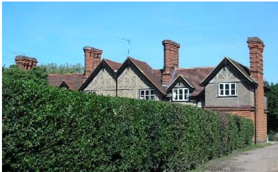
Griffins Wood Cottages
