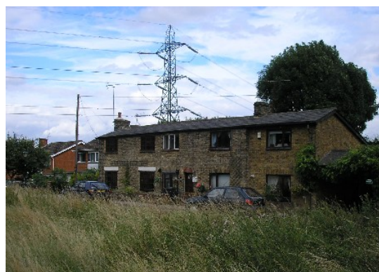
Electricity pylons outside the conservation area
