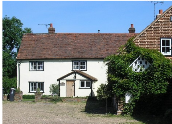
Ladderstile Cottage, Grade II listed
