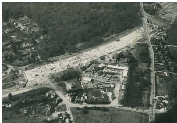
Construction of the M25 tunnel immediately to the south of Bell Common
