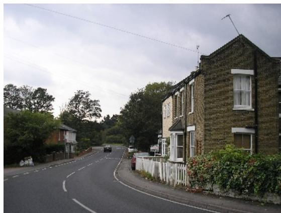
Area 3. Group of houses on Theydon Road
