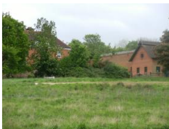
Little Copped Hall (left) with model farm building at Home Farm (right)
