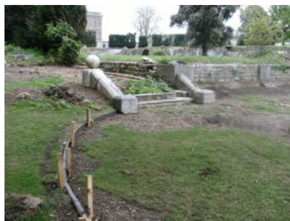
Garden restoration in progress
