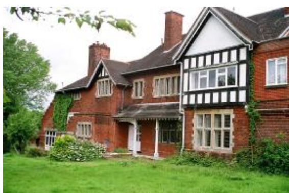
Griffins Wood House
