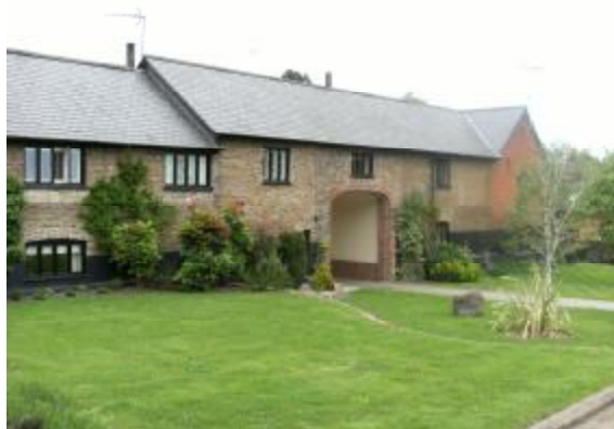
Nos. 1 & 2 The Hall Barns, Copped Hall
