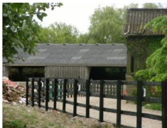
Disused former farm buildings at Home Farm
