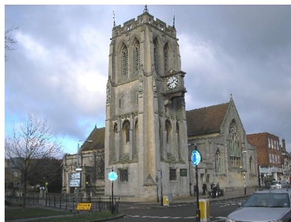
Setting of St John's Church with street furniture
