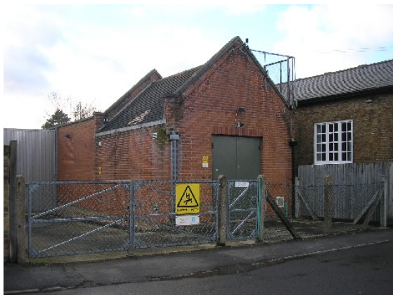
Electricity sub-station on Lindsey Street
