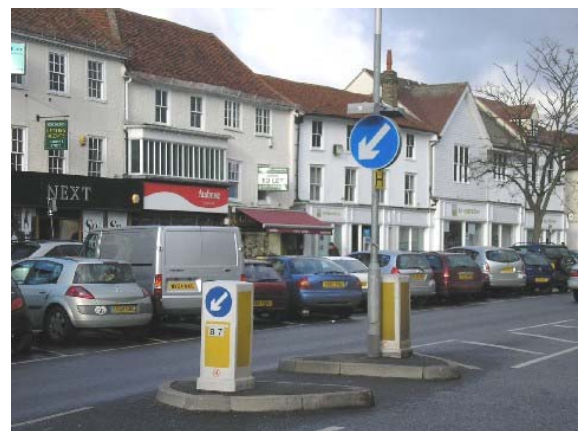
Road signs on the High Street that are out of character with the conservation area
