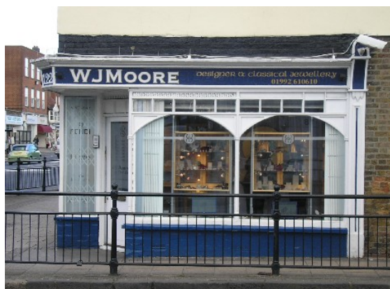
Traditional timber shopfront at 120 High Street
