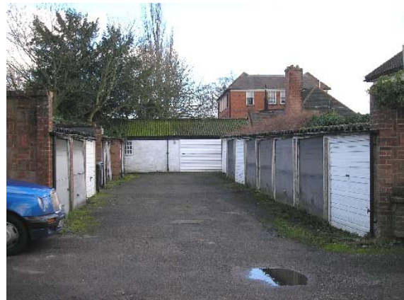
Lindsey Street lock-up garages
