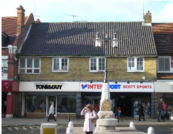
Continuous strip of fascias without subdivisions which looks out of place on a historic street
