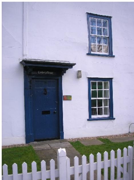
Sliding sash windows, decorative doorcase and picket fence on 98 High Street, Grade II listed
