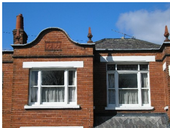
Red brick and slate on 9 Church Hill
