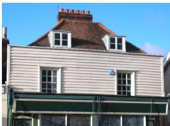
Weatherboarding and plain clay tiles on 269 High Street, Grade II listed
