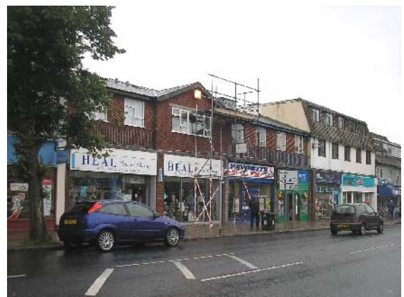
Some dominant deep fascias on shopfronts on the High Street
