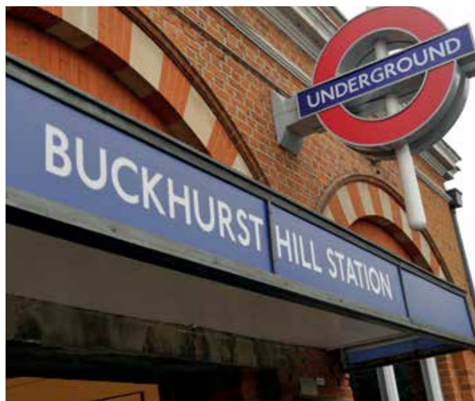
Buckhurst Hill Station
