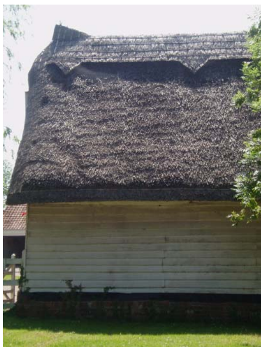
Weatherboarding and thatched roof on one of the barns belonging to Matching Hall
