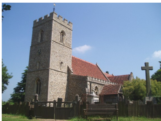
St Mary's Church, Grade II* listed
