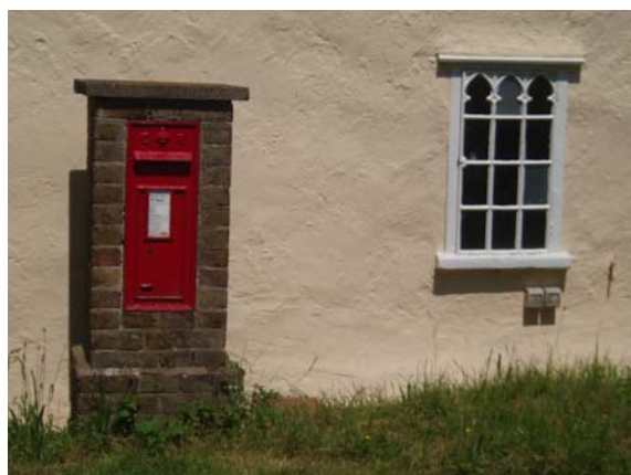
Red letterbox and cast-iron Gothic window on the Marriage Feast Room
