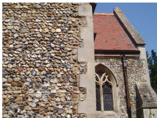
Flint rubble stone walls on St Mary's Church
