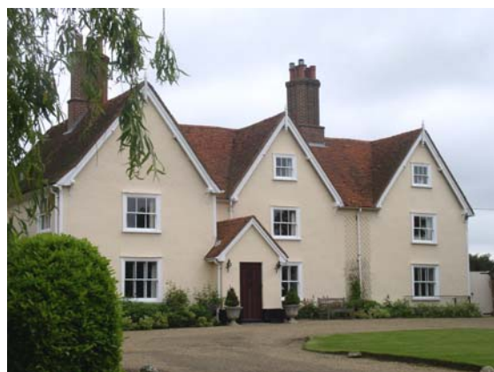
Matching Hall, Grade II* listed
