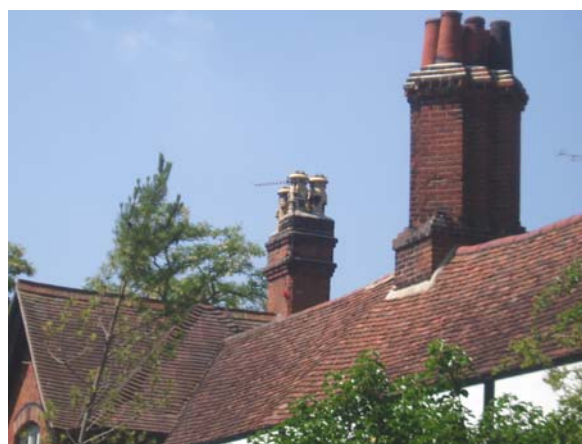
Plain clay tile roof on the Vicarage
