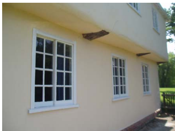
Horizontal sliding sash windows on the Marriage Feast Room
