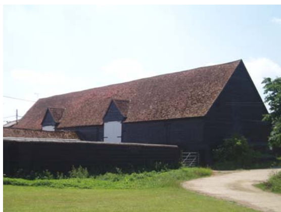
Timber-framed aisled barn, Grade II listed
