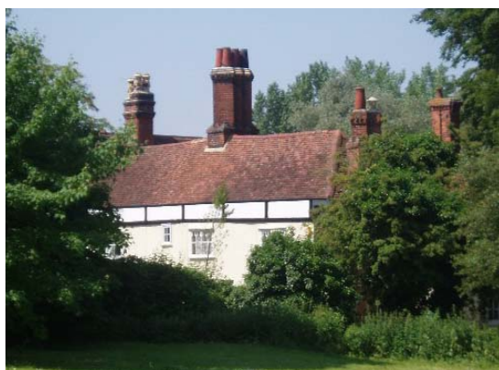
The Vicarage, Grade II listed
