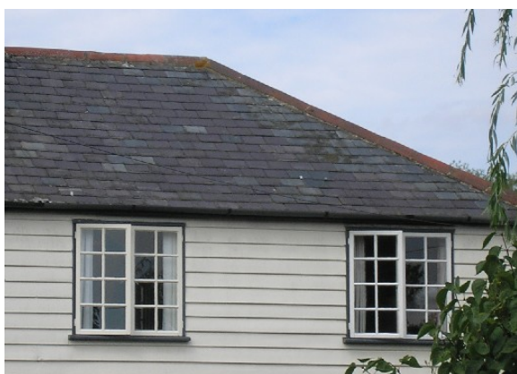
Traditional weatherboarding, natural slate and timber casement windows on Lilac Cottages
