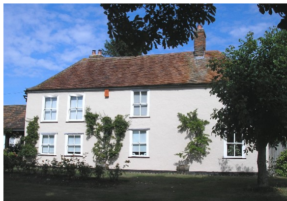
Albion House, Grade II listed
