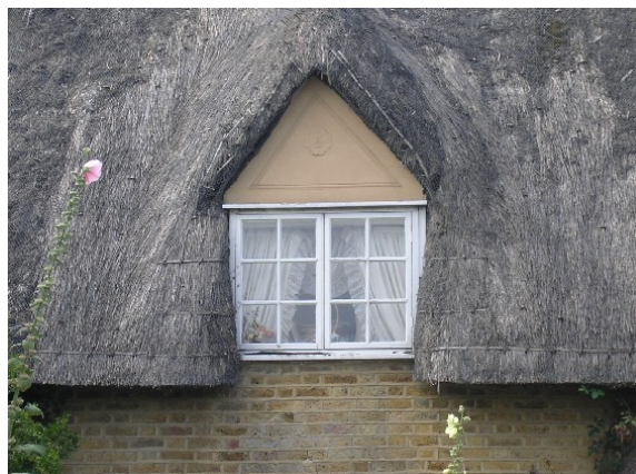
Yellow stock brick, decorative pargetting & thatched roof on Forge Cottage, Grade II listed
