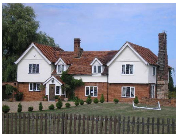
The Moat House, Grade II* listed
