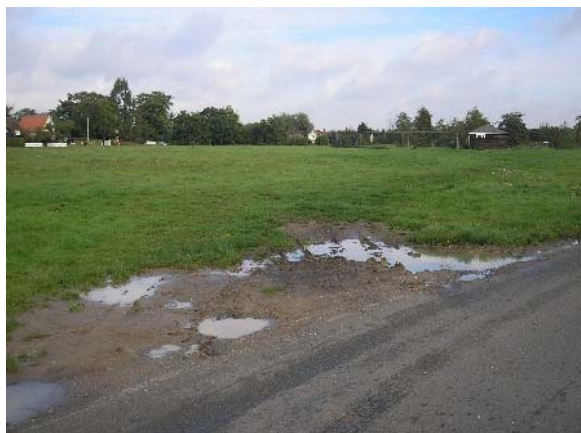
Edges of the green eroded by parking
