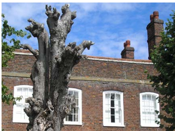
Early 18 th century sliding sash windows and red brick on The Limes, Grade II listed
