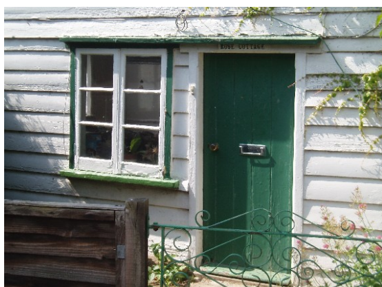
Weatherboarding and traditional casement window on Rose Cottage
