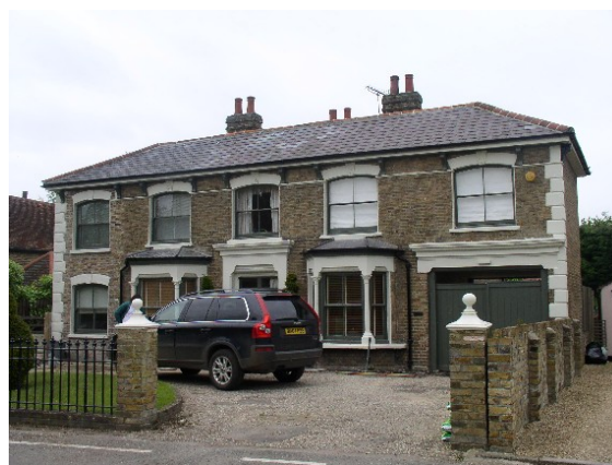
Sommerfield House, locally listed
