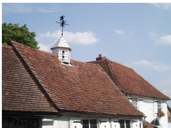
Traditional plain clay tile roof on Gainsborough Cottage
