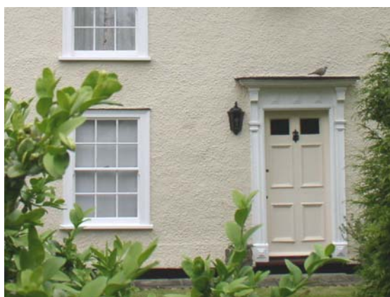
Decorative doorcase and sliding sash windows on Shetlocks Farmhouse
