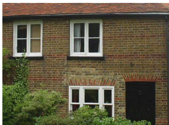
Decorative brickwork on Shetlocks Cottages
