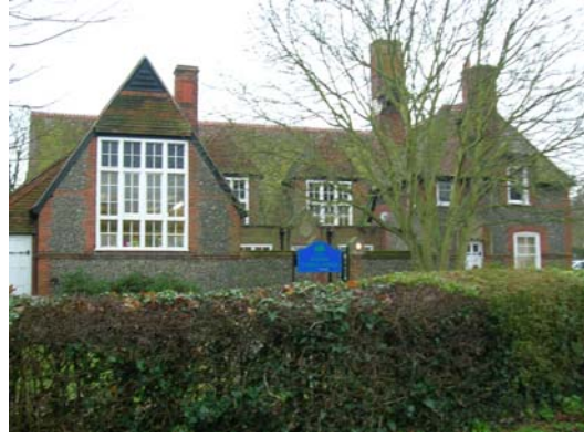
Roydon Primary School on Epping Road
