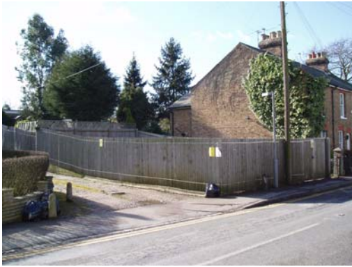
Electricity sub-station on Epping Road
