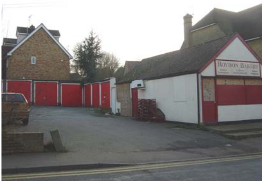
Roydon Bakery and lock-ups, Harlow Road
