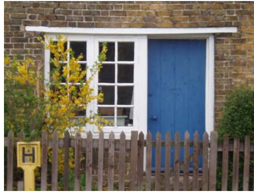
Early shopfront at 55-57 High Street
