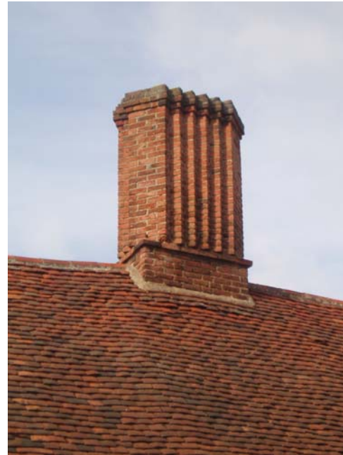
Decorative brick chimney and hand-made plain red clay tiles on The Niche, Harlow Road
