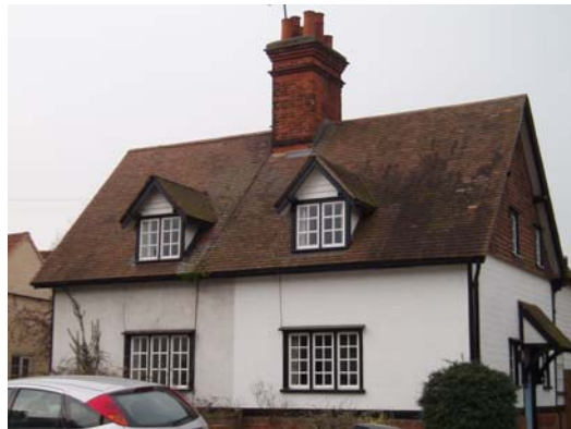
77 & 79 High Street, a locally listed building
