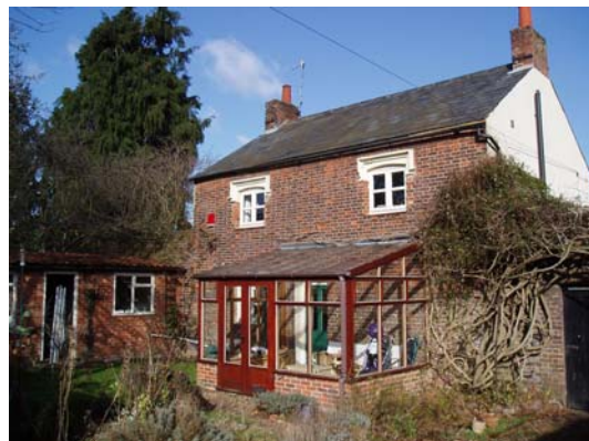
150 High Street, gardener's cottage of the former Roydon Lodge
