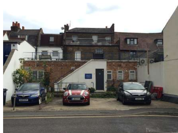
Unsympathetic 20 th century additions to buildings, Darby Drive (EFDC)
