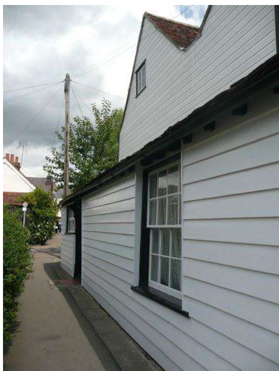
Weatherboarded cottage, South Place (EFDC)
