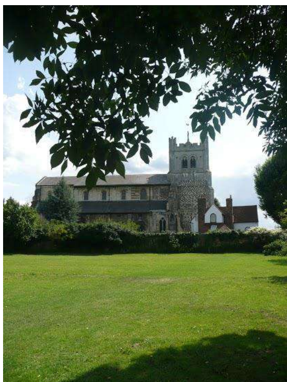
View of Church and vicarage from Abbey Gardens (EFDC)
