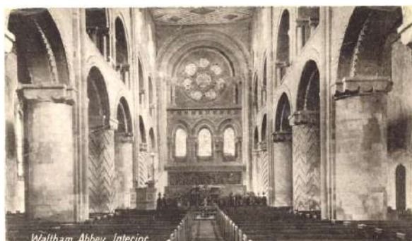
Waltham Abbey Interior Interior of Waltham Abbey Church (Old Waltham Abbey in pictures, K.N. Bascombe)
