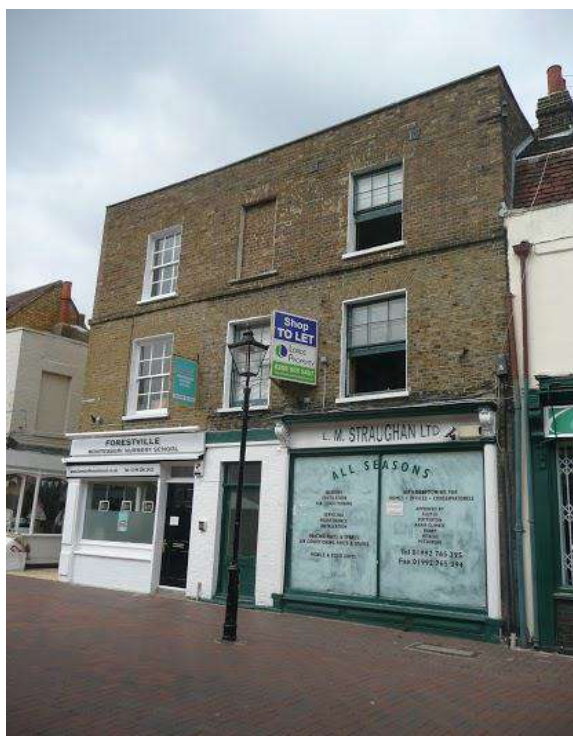
Vacant shops, Sun Street (EFDC)
