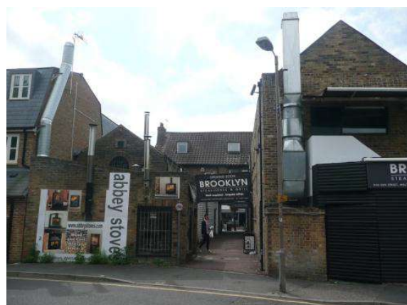
Unsympathetic alterations to buildings, Darby Drive (EFDC)
