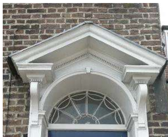
Hooded pediment door with fanlight (no. 16 Sewardstone Road) (EFDC)
