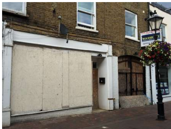
Vacant shops, Sun Street (EFDC)
