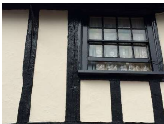
Traditional timber framing (EFDC)
