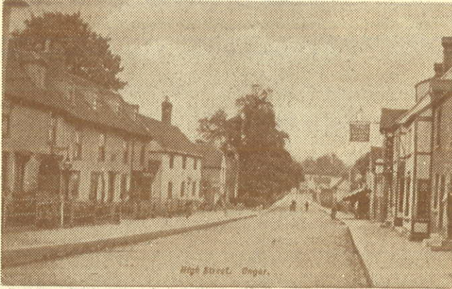
This view of the High Street, taken around the turn of the century, shows Livingstone Cottages on the left hand side. The ground floor of one of the cottages was removed to create the arched accessway through to the United Reformed Church which was built in 1833. Included in one of the cottages is a room in which the missionary and explorer David Livingstone spent some time as a lodger in 1838 before departing for Africa.
