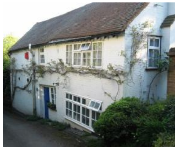
Kings Cottage, Kings Hill, Building of Townscape Merit
