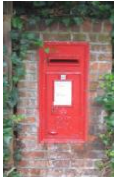
Post Box at the top of York Hill
