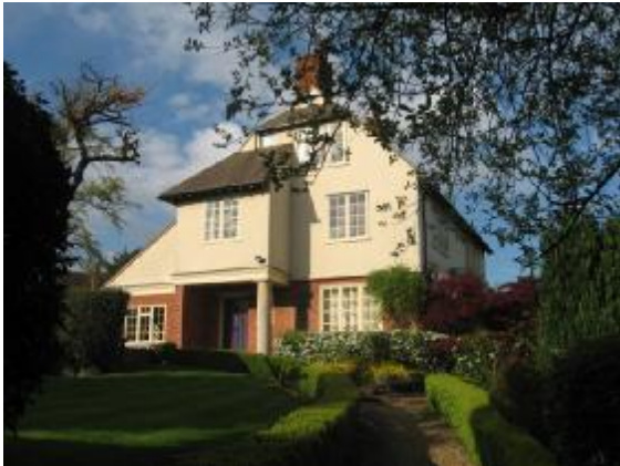
Woodberrie, features original casement windows, and part rendered brickwork
