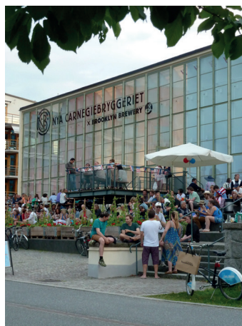
Re-use of a mid-century building as a brewery and bar in Hammarby Sjostadt, Sweden
