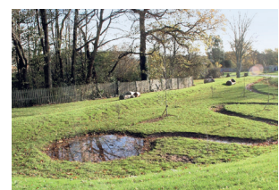
Attenuation ponds retain run-off and remove contaminants before draining into a water course.
