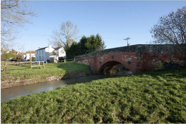
Main View of Moreton Bridge
