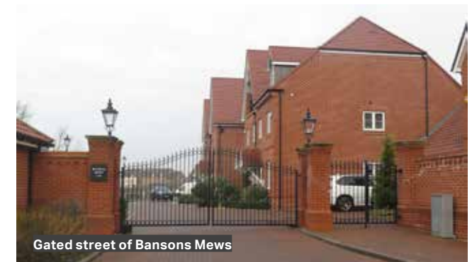
Repeating pattern of symmetrical pairs of semi-detached houses
