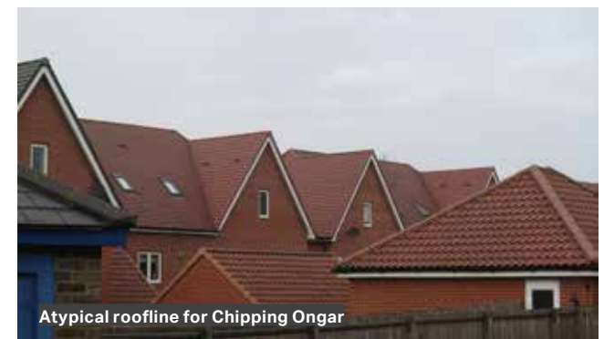
The varied roofline of the High Street
