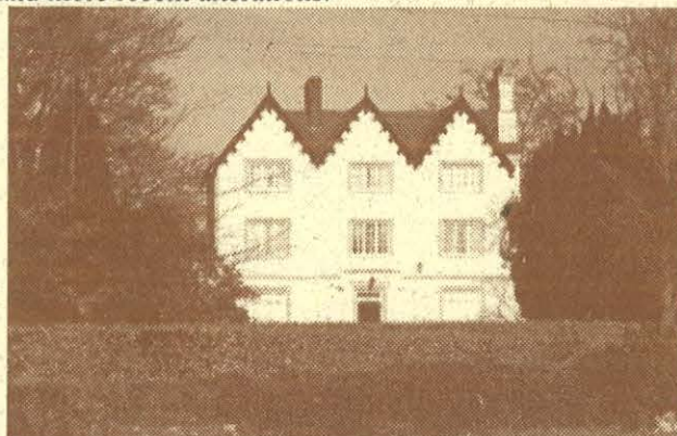
The photograph above shows the imposing gabled front elevation of Castle House, a Grade II Listed Building which dates from the 16th century. Although altered in c.1840, many original 16th century features survive including tie beams and panelling.
