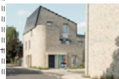
Goldsmith Street, Norwich Built to Passivhaus standards, needing little energy for heating and cooling.
