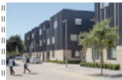
Virido, Cambridge Zero-carbon development of 208 homes, achieving Code for Sustainable Homes Level 5.
