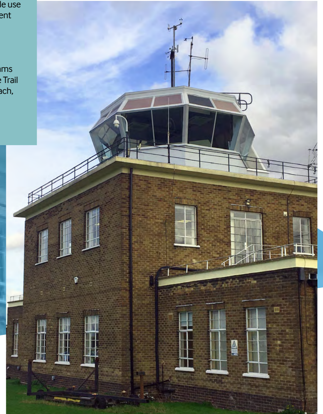
Existing Air Traffic Control Tower
