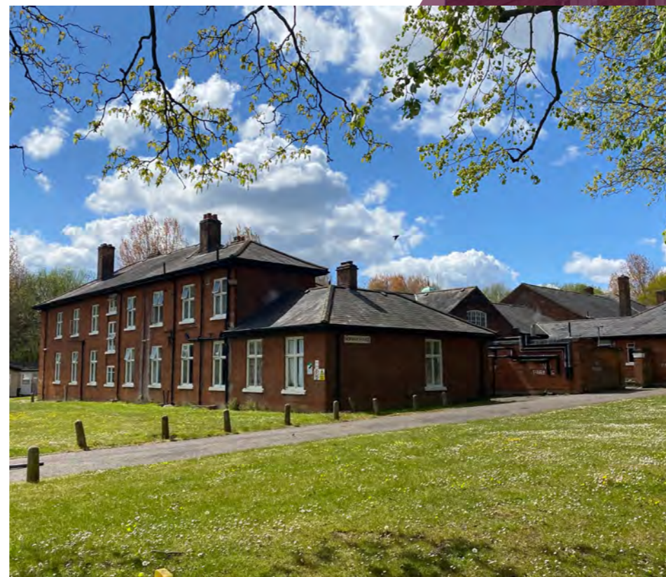
Norway House (former Officer's Mess)
