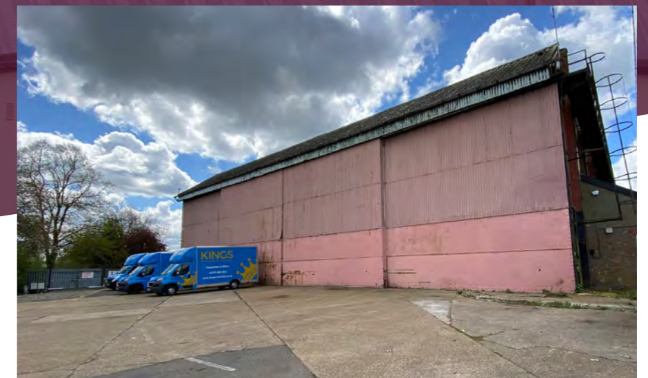
Existing Hanger 1 structure located within the southern part of the site
