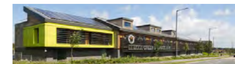
Filwood Green Business Park, Bristol – An example of an environmentally friendly employment development
