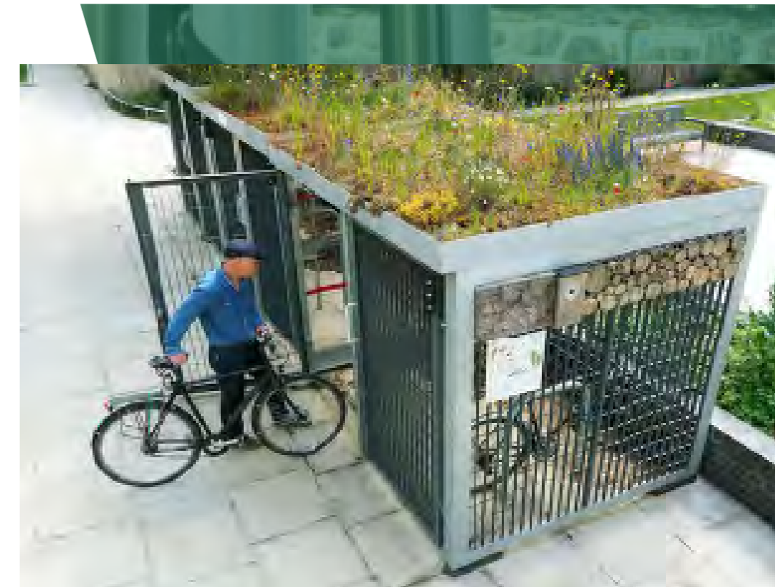
Cycle store with green roof
