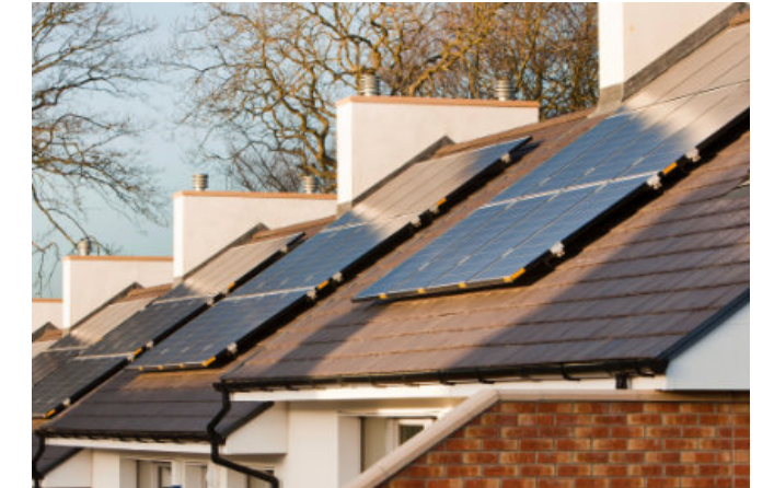
Photovoltaic cells used where suitable
