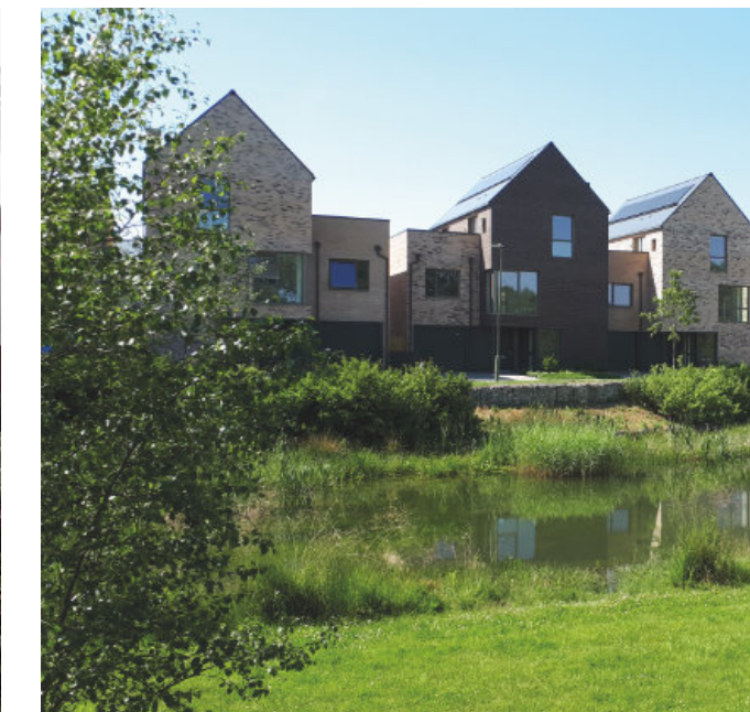
Housing set around SuDS pond
