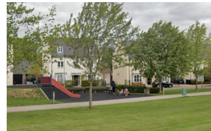
Guilden Park in north Harlow achieves an open space that is active (children's play space) and overlooked by surrounding residential properties.
