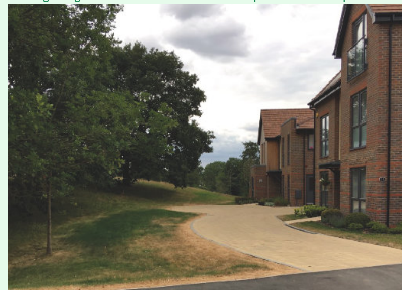
Housing facing on to woodland tree belt
