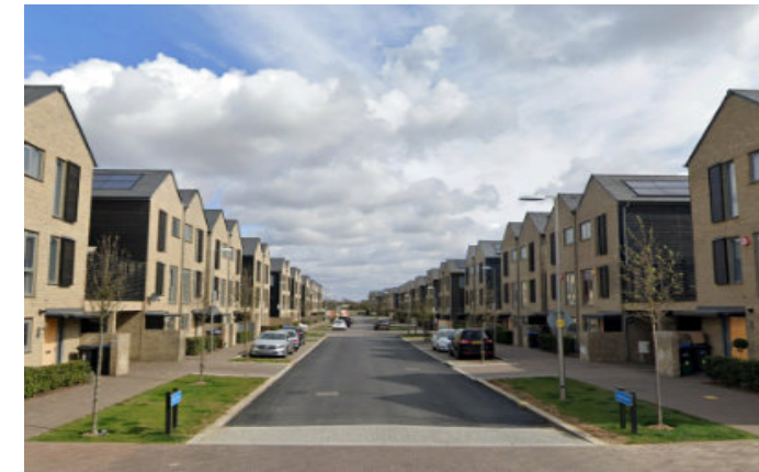
New Hall (phase 2) achieves a consistent and strong street character, with a mirrored architectural style down both sides and a sense of enclosure.
