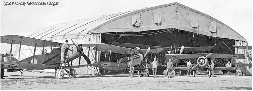
Typical six-bay Bessonneau Hangar
