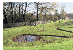
Attenuation ponds retain run-off and remove contaminants before draining into a water course.
