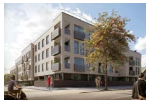
Tallack Road, Waltham Forest, London Large-scale communal Air Source Heat Pump to feed ambient temperature heat network
