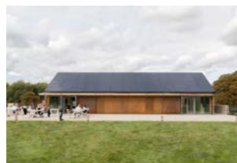
Cassiobury Park, Watford Multi-purpose community hub, designed with minimal energy consumption. It won the Most Sustainable Construction award at the 2018 Building Futures Awards.
