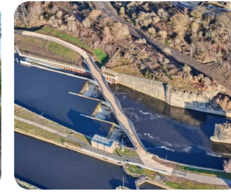
Knostrop Weir, Leeds | Flood Management Provides three new pneumatically moveable weirs that can be lowered to let floodwater discharge quickly downstream.
