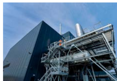
Millerhill, Midlothian Residual waste recycling and energy recovery facility
