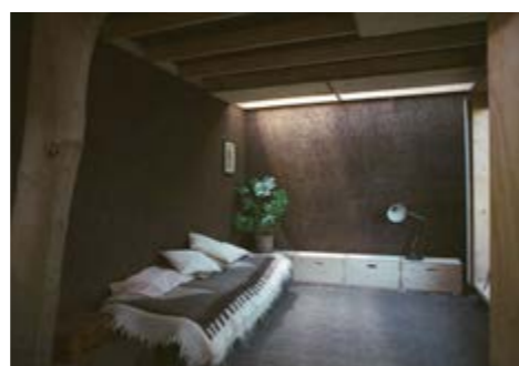
Cork Housing, Studio Bark A garden building made almost entirely out of cork, constructed as a building that can be completely recycled, reused or composted.
