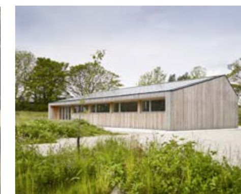
Argal Workshops (Gluckman Smith) A Cornish former farmstead, previously derelict, was transformed into rural workshops for a local furniture and product designer, to Passivhaus standards, making a new working community for the area.
