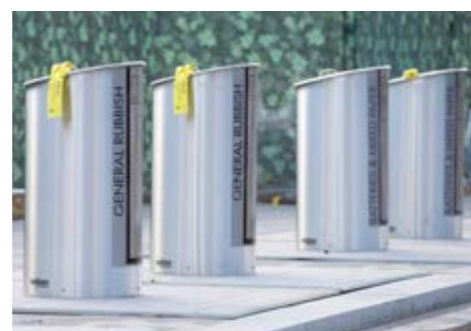
Eddington, Cambridge Underground chutes replace thousands of traditional wheelie bins in an innovative waste disposal system
