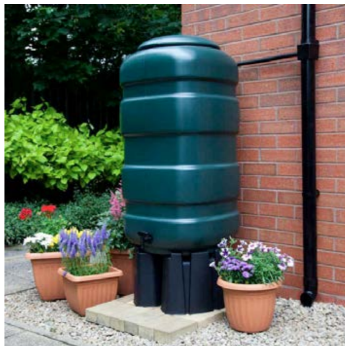
Example of domestic water management; water butts A water butt is essentially a large container used to capture and store rainwater. When attached to a downpipe, the water butt collects the rainwater that lands on the roof of a building so it can be used later. It is this time of year, when rainfall has been scarce, that water butts become really useful.
