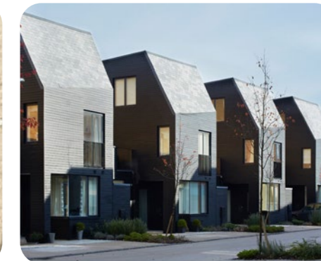
Newhall, Harlow Being highly sustainable with consideration for long-term energy use and incorporating measures to reduce energy use in properties
