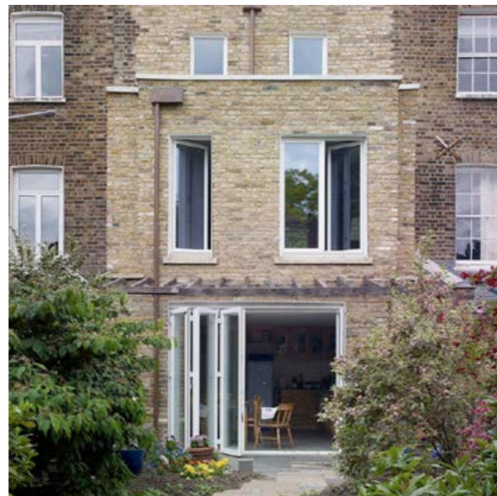
80% House (London) by Prewett Bizley Architects An extension to a townhouse that includes living, cooking and dining spaces. A rooftop extension adds a third bedroom-cum-study. The house achieves an 80% reduction in CO2 emissions, primarily by incorporating high levels of insulation and air tightness. Fresh air is supplied by an MVHR system. A photovoltaic array on the roof with a provides a little over half the annual electricity requirement.
