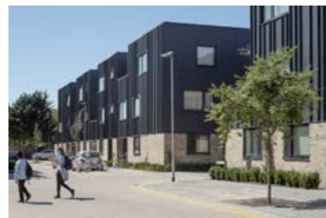
Virido, Cambridge Zero-carbon development of 208 homes, achieving Code for Sustainable Homes Level 5.
