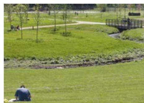
Ladywell Fields, Lewisham (SuDS) Designed to create more sustainable drainage and reduce flooding, the river channel was modified to create a naturalistic setting incorporating backwaters and wetlands.
