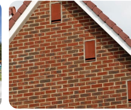
Ecology in Architecture: Barratt Homes A progressive approach to wildlife-friendly housing, with 'Swift Bricks' built into homes.
