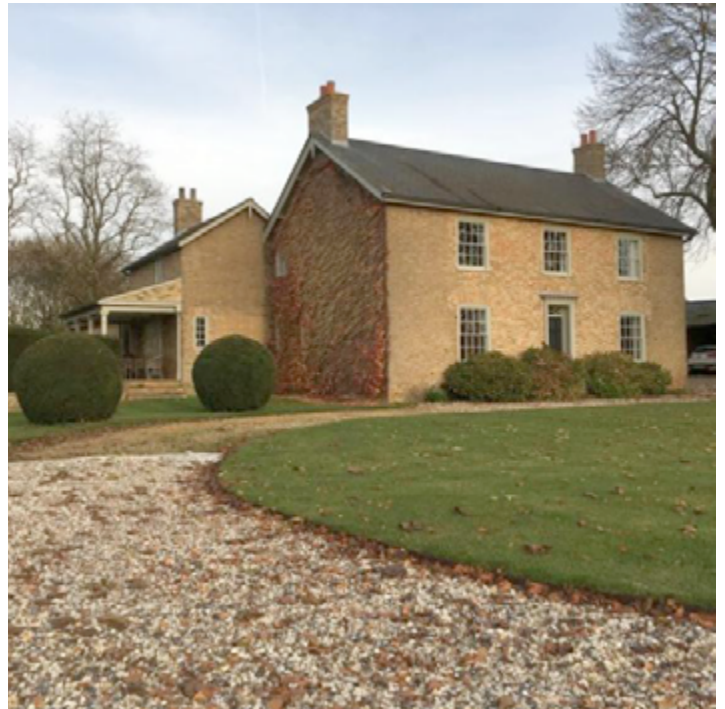
1860s Farm (Huntingdon), pump by Finn Geotherm
