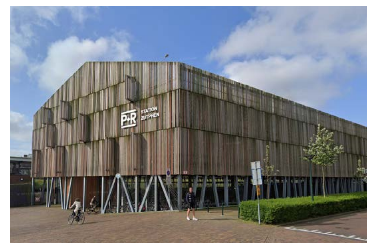
Example of remote parking barn in Zutphen, Netherlands by MoederscheimMoonen Architects.
