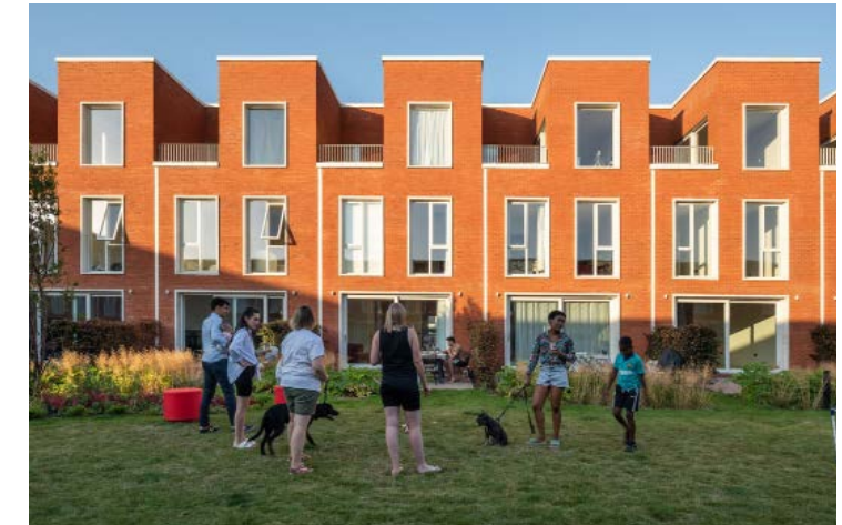
Broken terrace with terraces overlooking a shared garden. Brick House, Birmingham, by Howells
