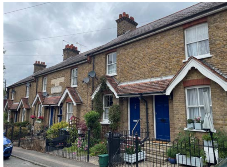
Articulated windows on Oddfellows Terrace, Old Harlow.
