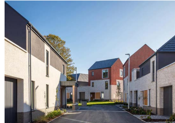
Marker house at Wilkinsons Brook, Tyrellstown, Ireland by Proctor and Matthews Architects.
