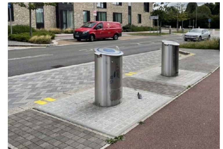
Underground refuse and recycling system, Eddington, Cambridge.
