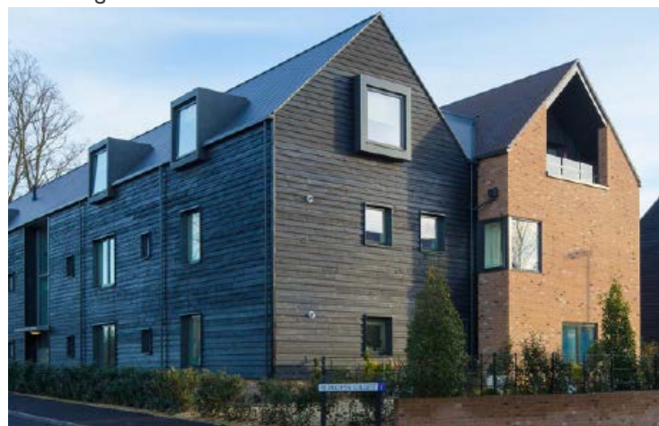
Apartment block form integrated with housing, The Avenue, Saffron Walden, by Pollard Thomas Edwards.
