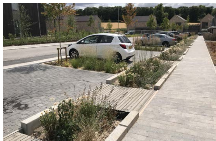
Attractive and functional on-street parking court at Loveden Fields, Hampshire by John Pardey Associates and BD Landscape Architects.
