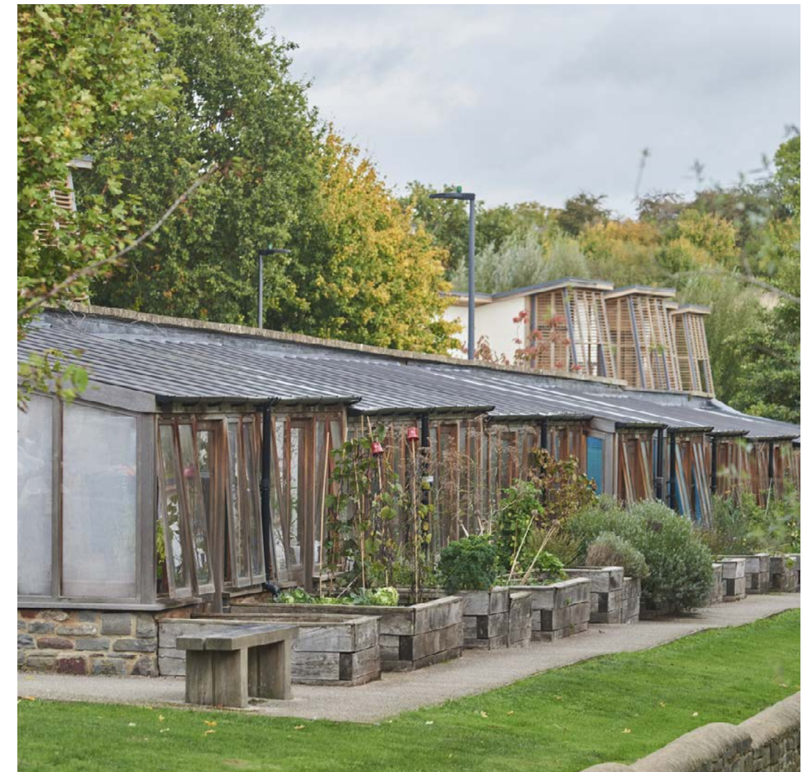
Shared greenhouses and beds at Hanham Hall, Bristol, by HTA Architects.
