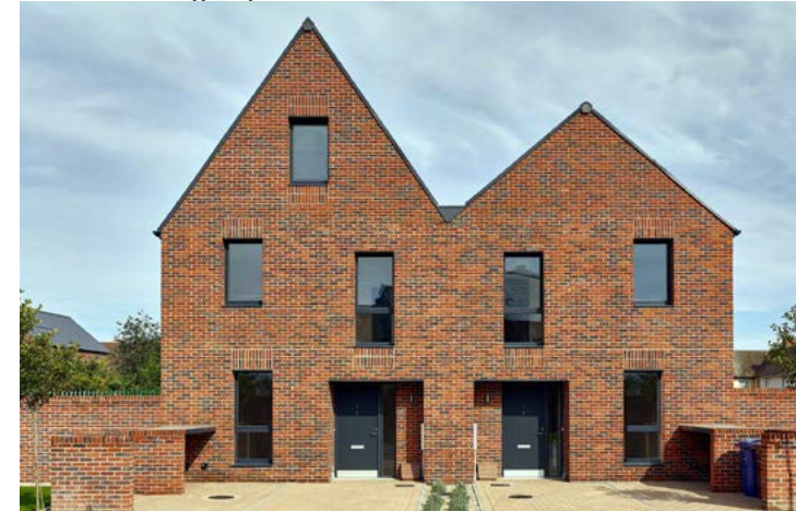
Compact semi-detached houses to maximise overlooking at St Chads, Tilbury by Bell Phillips Architects.
