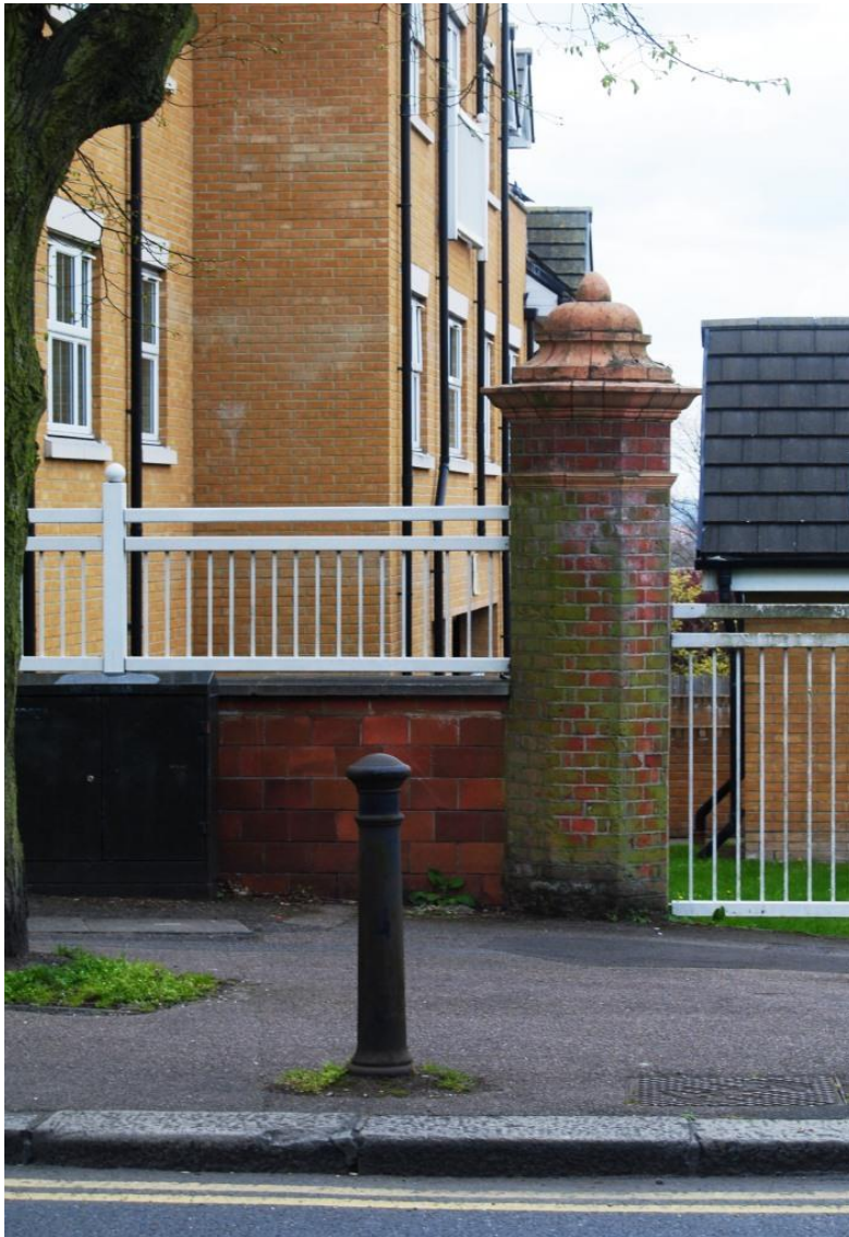
Figure 25: Wall and pier of now demolished Victorian reservoir
