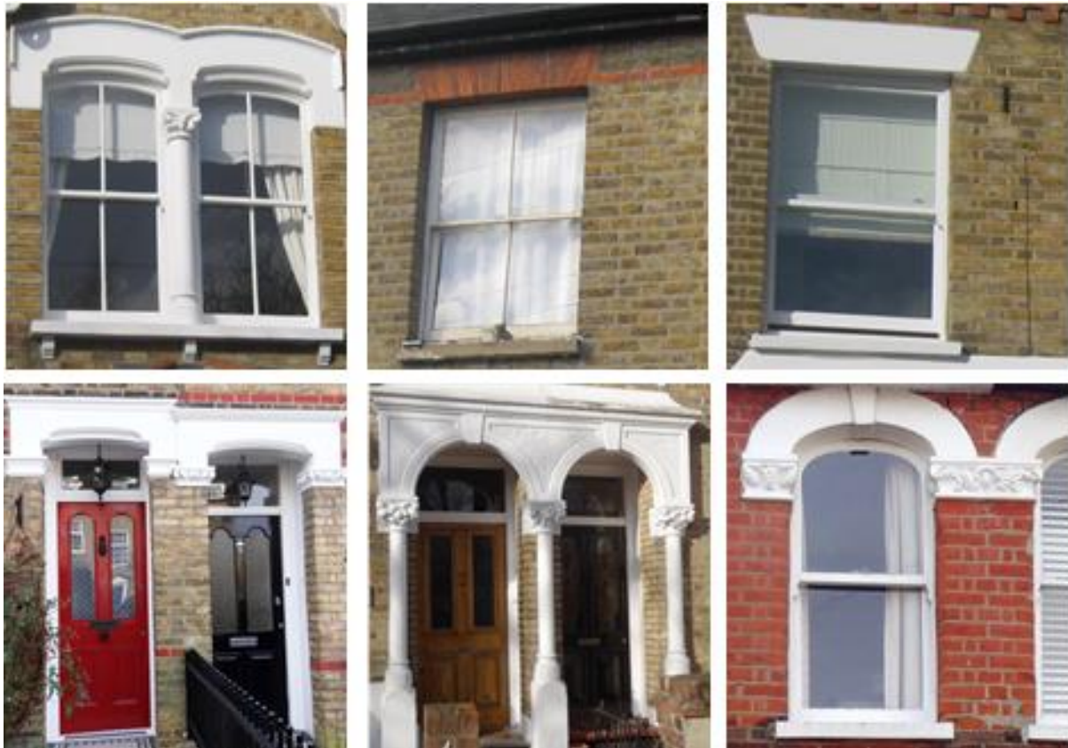
Figure 36: Timber windows and doors (historic and replacements)
