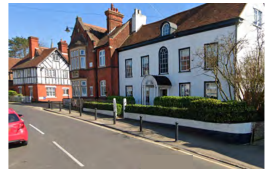
Mostly 2 storeys - some with attic rooms
